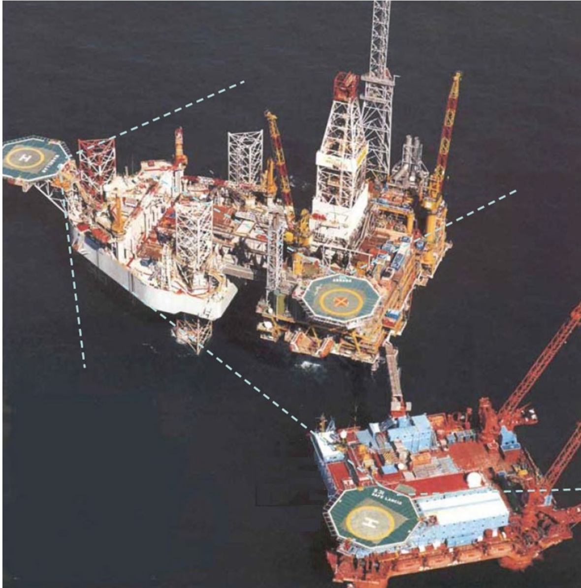
Figure 3: A temporary combined operation showing relative position of each helideck 210° sector
